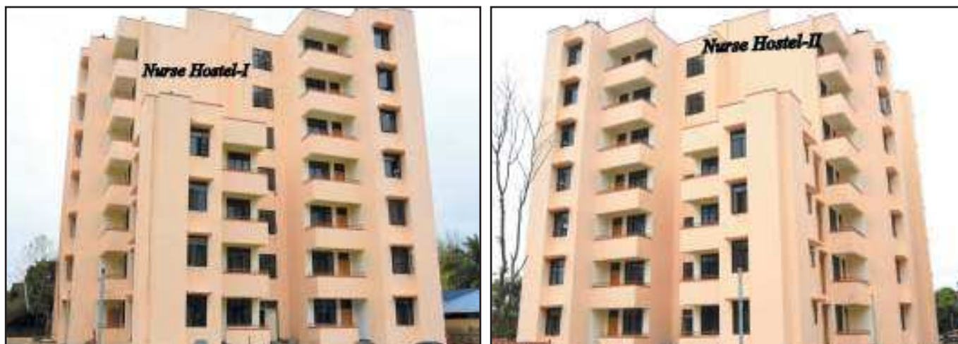
Infrastructure Development Work
